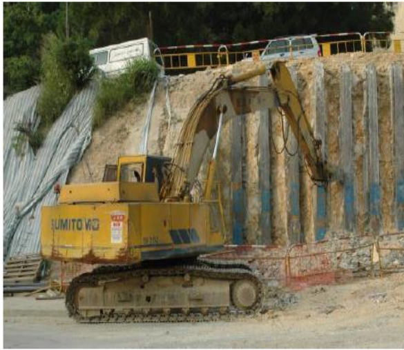
Power Drill (Breaking machine)
