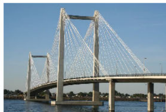
Cables support their loads in tension.
