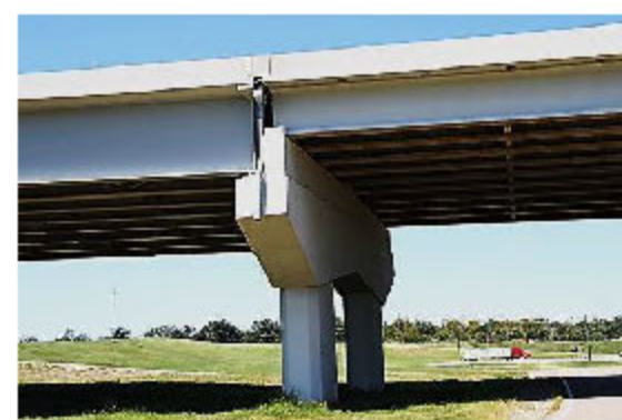
The prestressed concrete girders are simply supported
