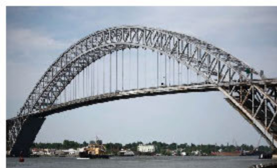
Arches support their loads in compression
