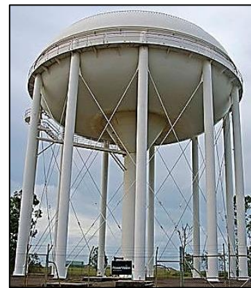
Columns as supports & compressive member in towers
