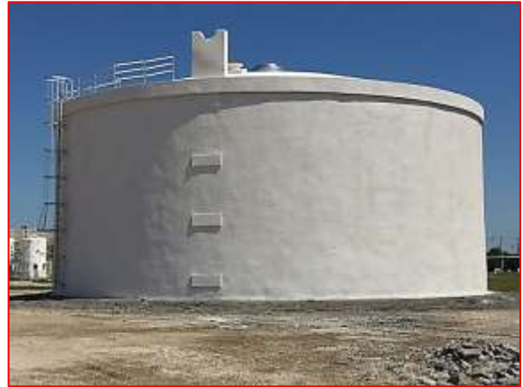
CIRCULAR RESTING ON GROUND TANK
