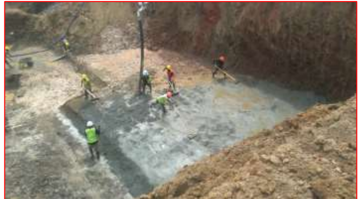
Cast the blinding concrete
