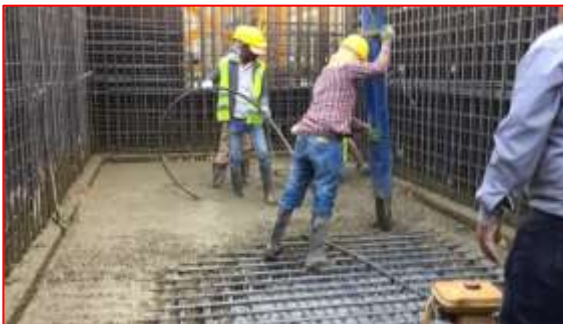
Cast of concrete
