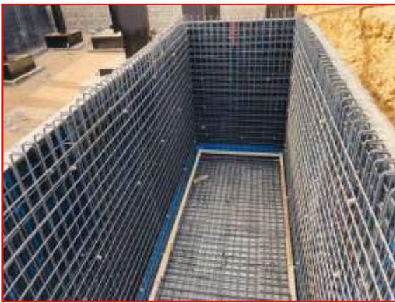
Reinfroced the wall and base
