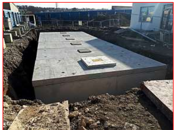
RECTANGULAR UNDERGROUND TANK
