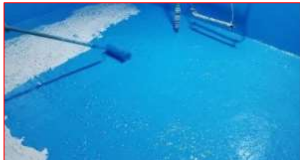
Lainding by using the suitable materials
