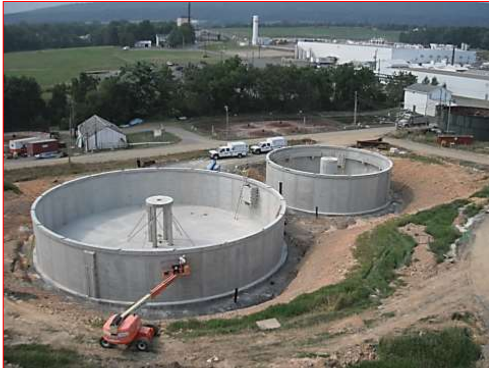
Case one. Wall not monolithic with the base.
