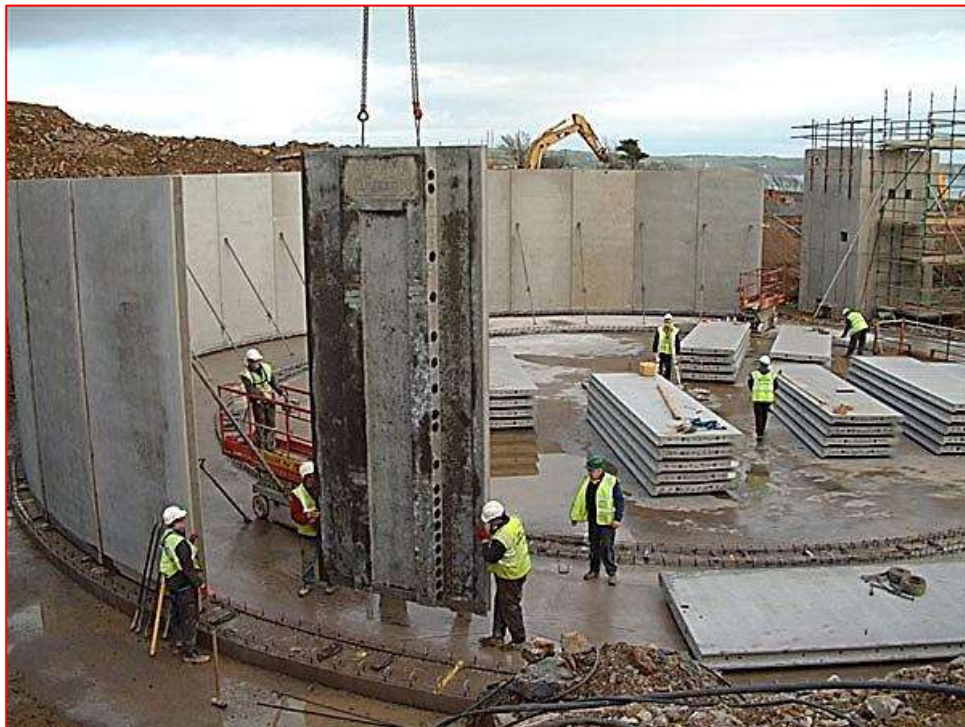
Case one. Wall not monolithic with the base.
