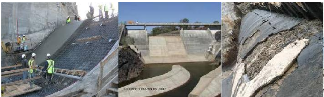
Cavitation effect on the spillway crest
