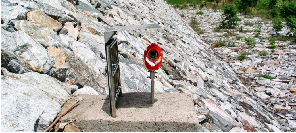
Automatic multi-purpose dam deformation monitoring system
