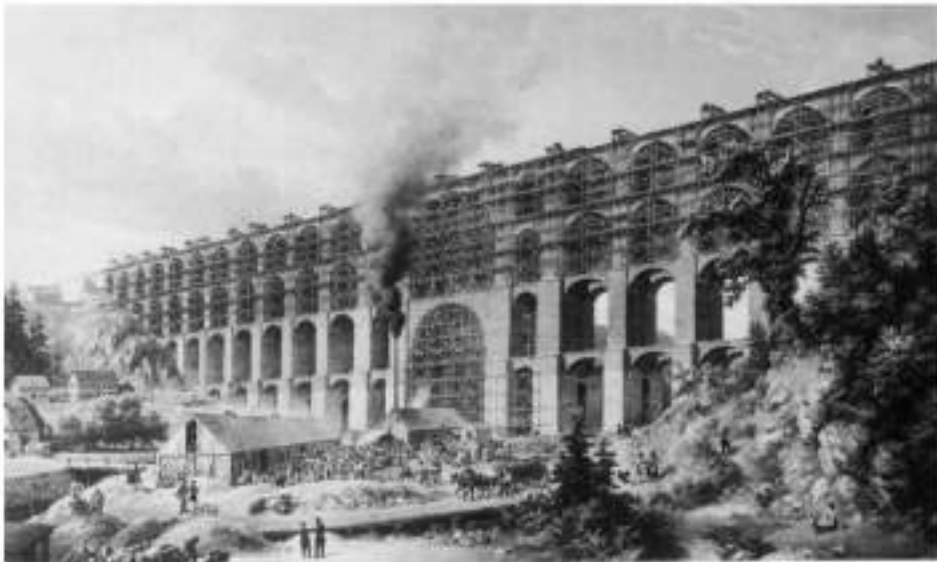
Göltzsch Viaduct around 1850 [Conrad & Hänseroth, 1995, p. 762]
