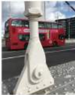
typical "pin supported" connection (metal) (a)
