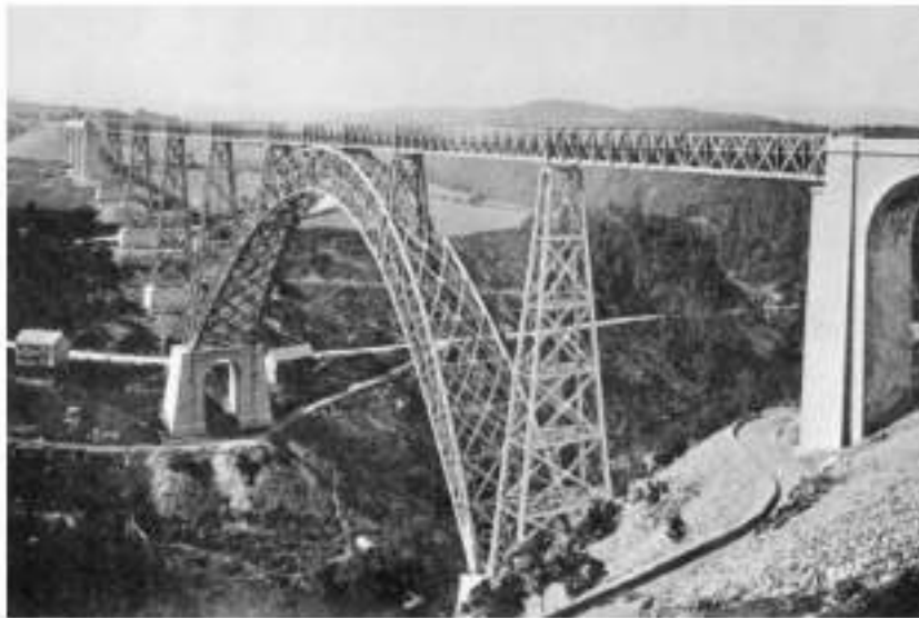
The Garabit Viaduct shortly after completion [Eiffel, 1889]
