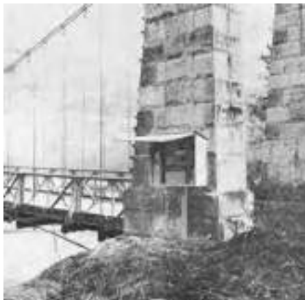
Fig. 4.5 Bubble Gauge Installation— Telemnip (Courtesy: Neyrtec, Grenoble, France)
