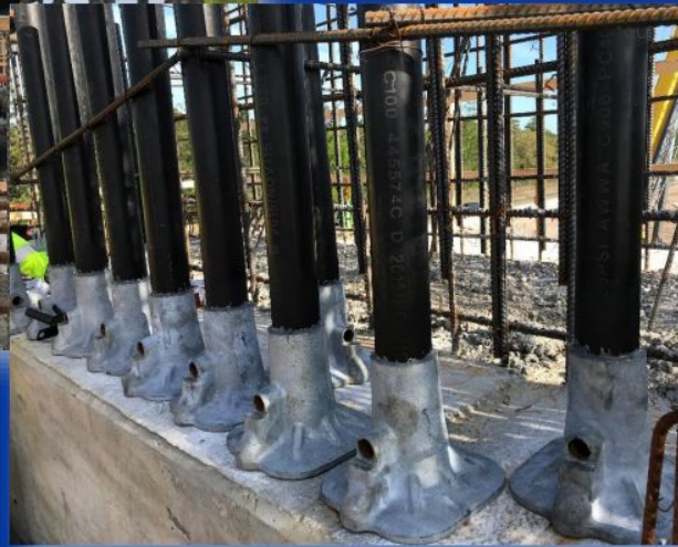
VSL PT anchorage for flexible filler
