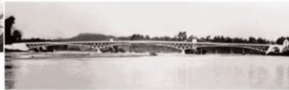
Fig. 1. Le Viaduc Bridge across the Allier River, France (1910-1911). Spans were 222 - 218 - 223 ft (67.5 - 72 - 67.5 m). This bridge incorporated the first use of thrust by jacks at midspan for decentering and also compensating for concrete creep and shrinkage. (Designed and built by Eugene Freyssinet.)
