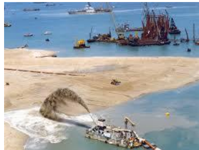
Reclaimed land, http://www.jandenul.com/en/activities/dredging-and-marine-works/land-reclamation-and-beach-replenishment
