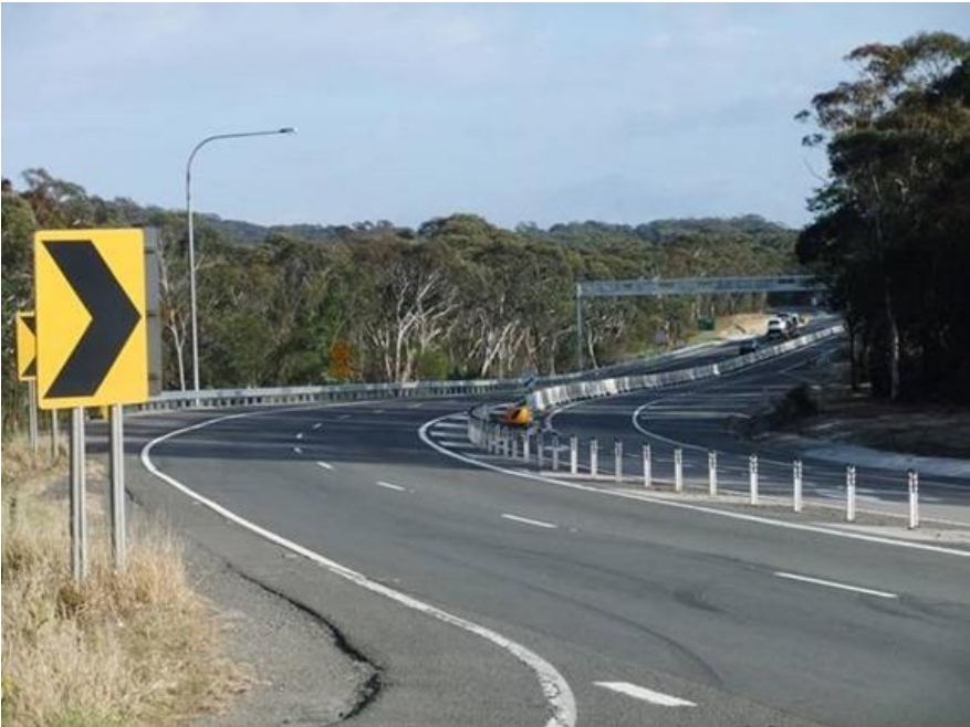
Figure 1.15: Highway alignment in three dimensions
