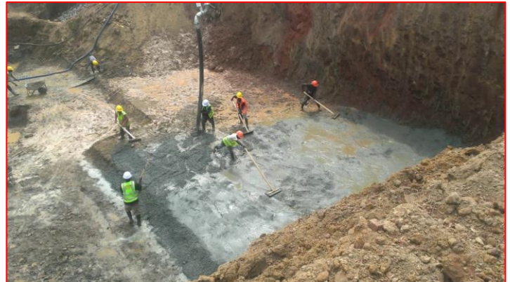
Cast the blinding concrete
