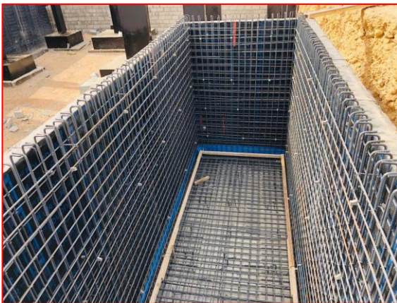
Reinforced the wall and base
