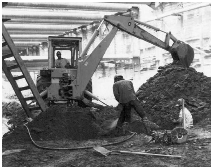
Figure 5.3 Braced cut in the construction of Washington, D.C. Metro, May 1974 (Courtesy of Ralph B. Peck)
