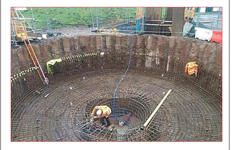
In this method some portion of the tank of the base acts as a cantilever & some load at the bottom is taken by the cantilever effect.
