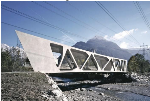
Figure 3.4-8: Concrete trusses with members under tensions.
