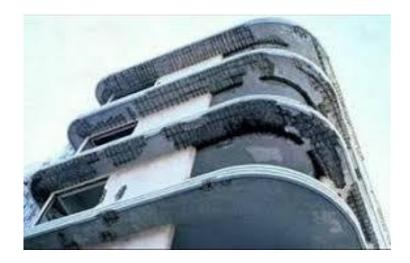
The thickness of reinforcement cover is an important factor controlling the
